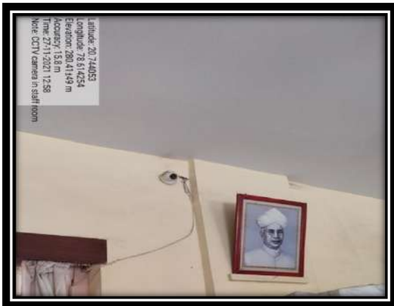
CCTV camera in staffroom
